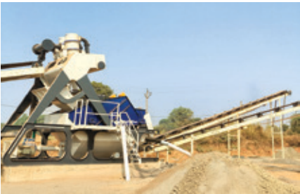
Rajasthan | Dewatering Screen
