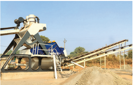
Rajasthan | Dewatering Screen
