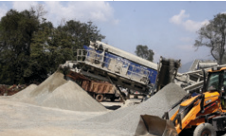
Jammu and Kashmir | Track Inclined Screen
